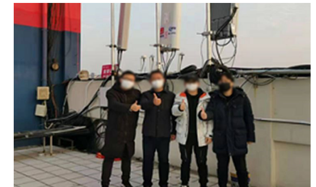
Figure 2: 5G + Wi-Fi network construction for Leishenshan Hospital
