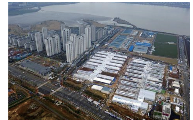
Figure 3: Live broadcast of Huoshenshan Hospital construction
